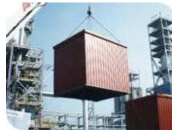
While the argument can be made that in some industries, a bottom lift design is the established standard for a prefabricated building design, that doesn't mean that it's always the best method for *your* prefabricated building. Cost and Convenience can play a significant role in determining the lifting method of a building.
